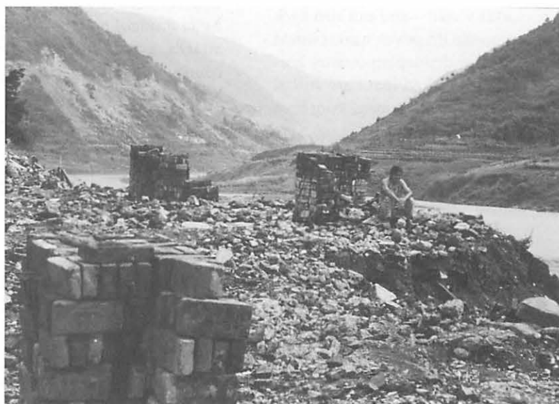
A worker sits on the ruins of a demolished building in an area to be flooded by the Three Gorges Dam reservoir.
