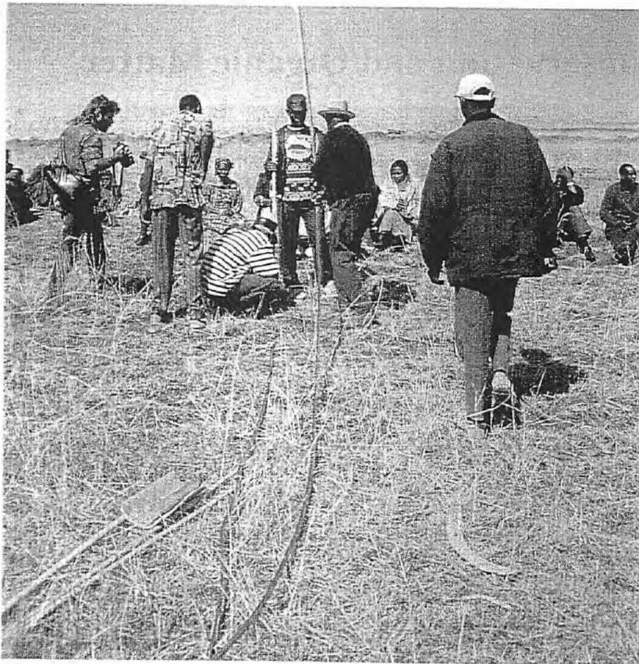
Hose-level construction in progress.
