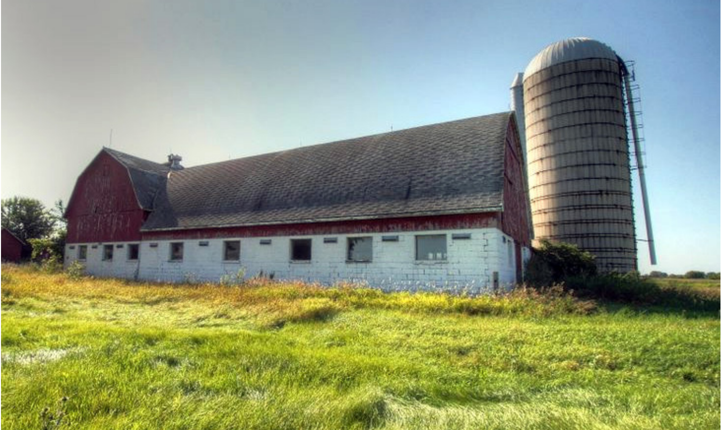
Abandoned Dairy Farm Barn. Photo by Ryan Schmitz (CC BY 2.0)
